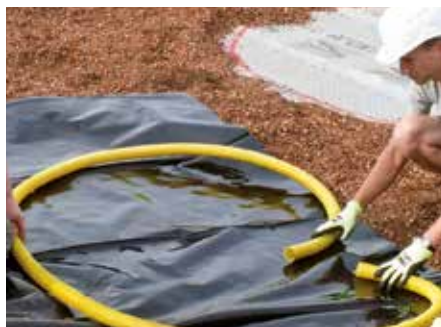
Temporary water areas created using drainage pipes and sheeting.
