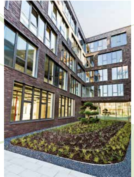
Inner courtyard equipped with a Stormwater Management Roof build-up on top of an underground car park in Ratingen, Germany.
