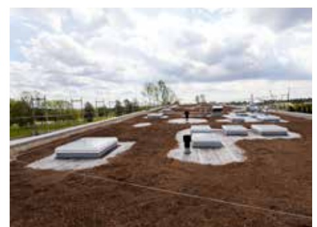
Installed system substrate "Rockery Type Plants".
